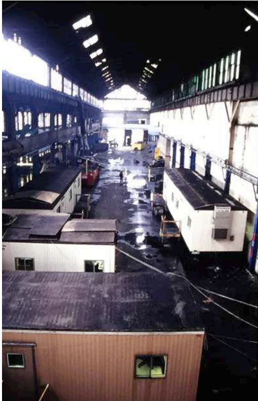
Trailer in the Highbay for Temporary Working Space During Construction
